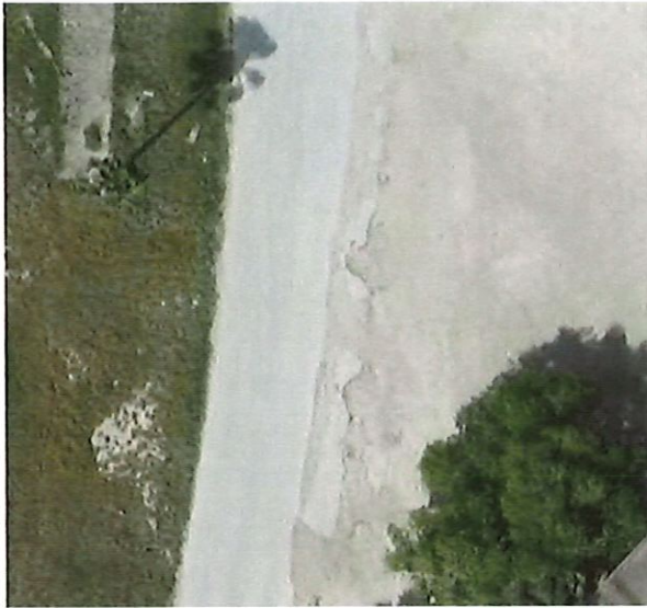
Figures 7 & 8. Examples of a street classified as being in "Poor" condition. Here there is a significant level of cracking and potholes with a higher level of separation between the cracks.
